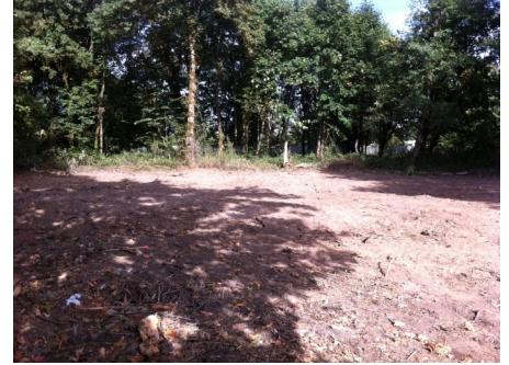
Chinook Park site cleared of underbrush, debris, and unhealthy trees.
