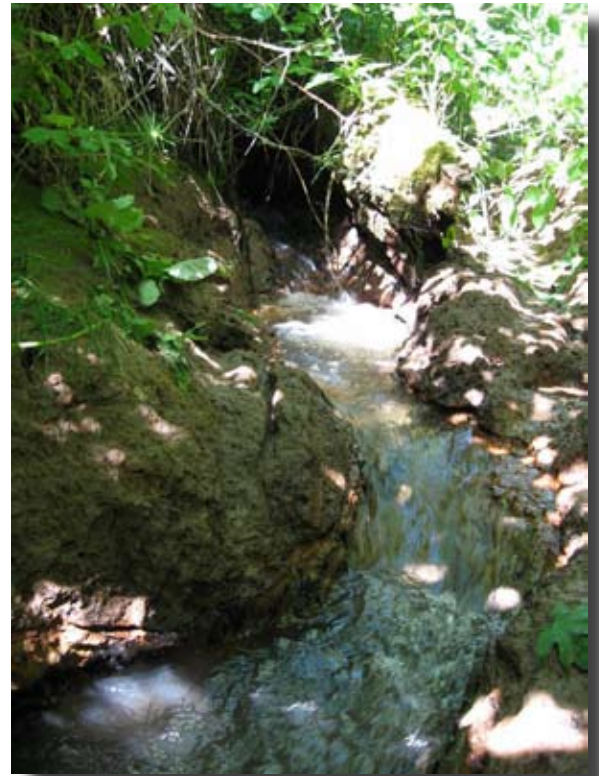
Channel erosion in project area.
