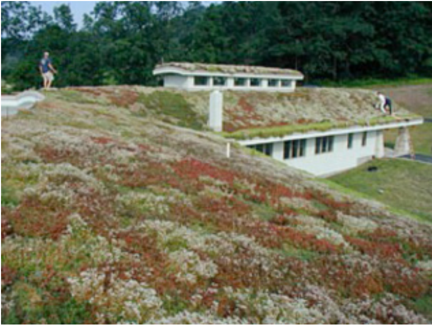
■ FIGURE 4-5. Green Roof
