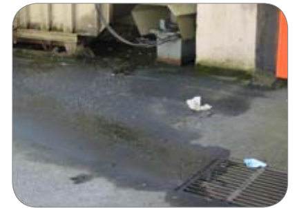
Pollution draining to stormwater system
