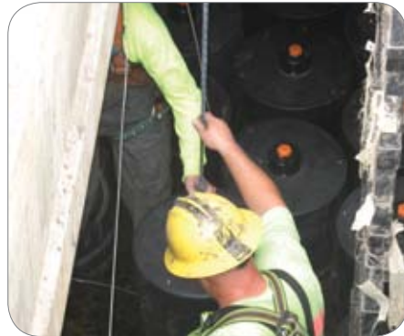
Replacing stormwater filters
